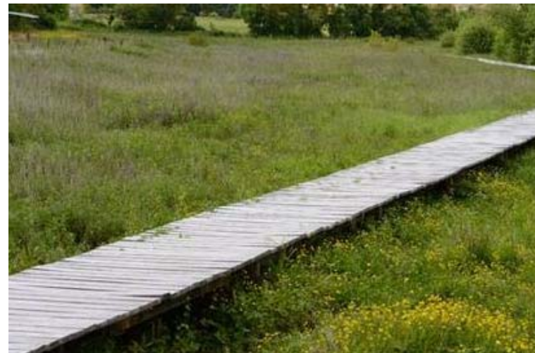
Link between Area A and C- Elevated Walkway. Finish level to be 150 mm above adjoining planted area.
