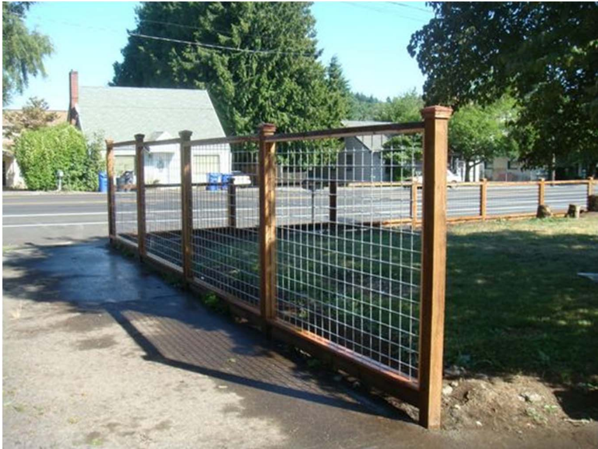
Timber Fence Zone 4 Dog Area- 1.6 m high Clifftop- 1.8m high
