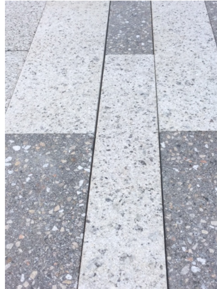
Acheson & Glover paving is has been selected for the plaza area and the central junction point in the park. It is a permeable paving option, slip resistant, frost resistant and suitable for heavy pedestrian traffic.
